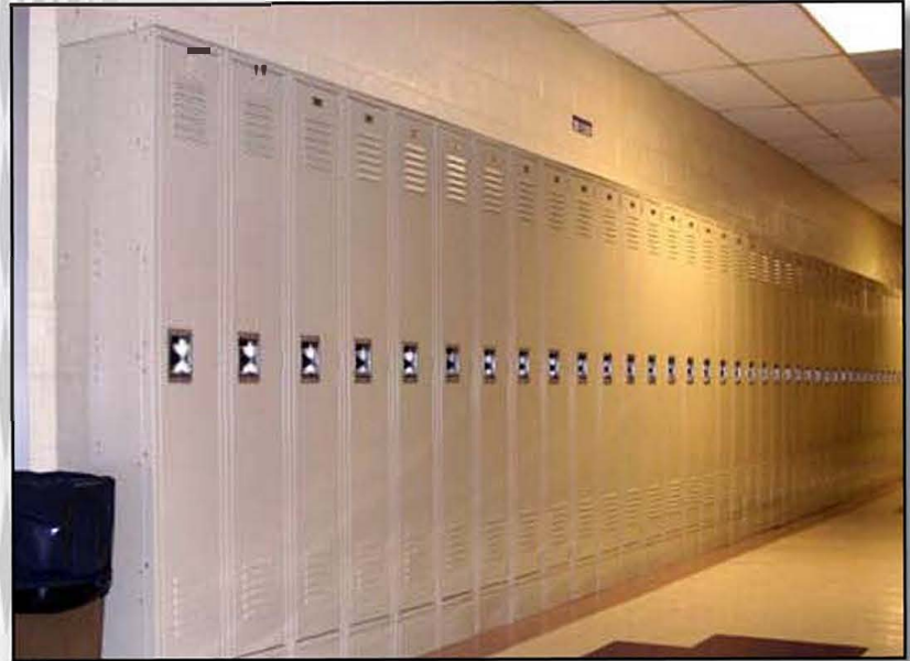
TYPICAL CORRIDOR LOCKER INSTALLATION WITH SLOPING HOOD
